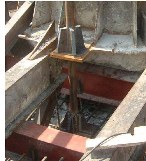
Lower connection with foot plates and welded web plates
