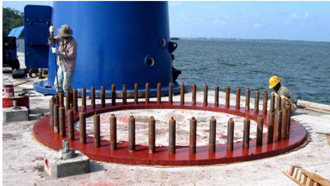
Upper connection with threaded rods
